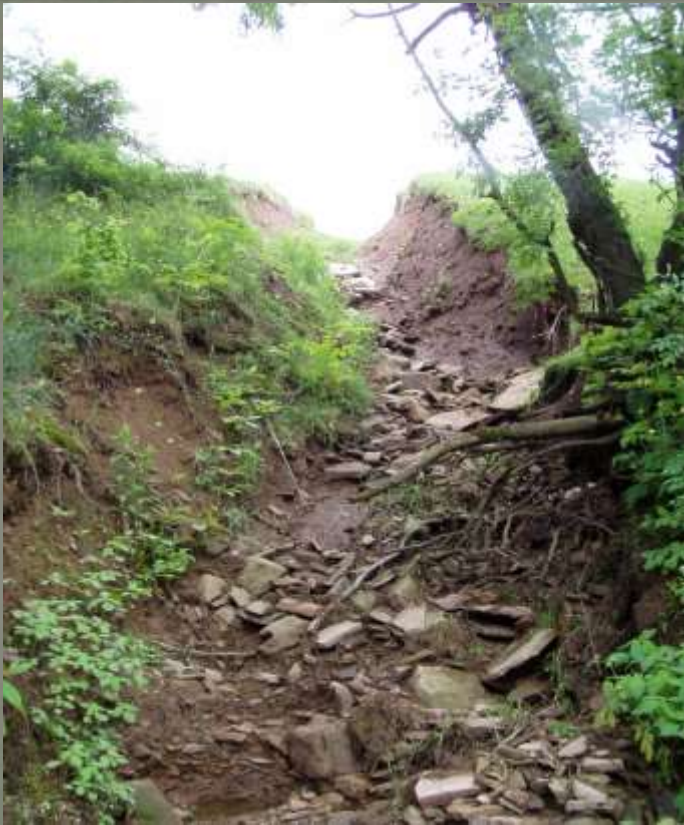
Ditch caused by diversion outlet
